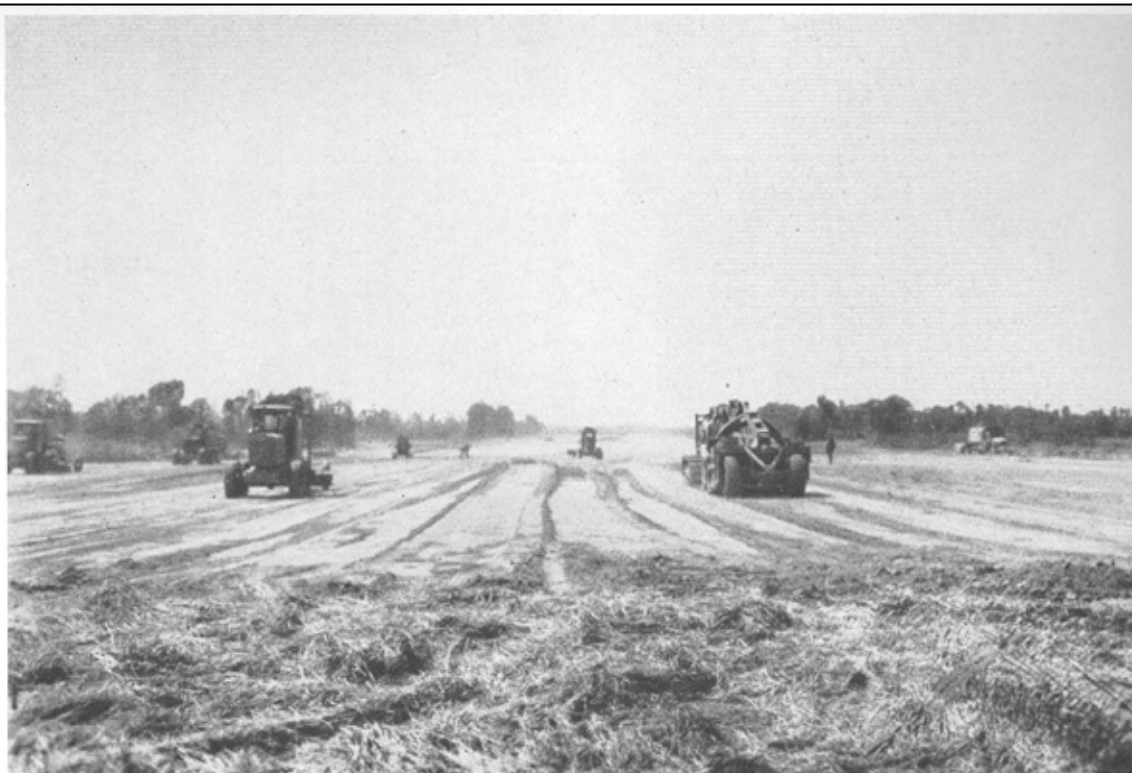
Heavy equipment grading on the runway extension at the second airfield. Deux-Jumeaux, A-4, Normandy, June 1944
