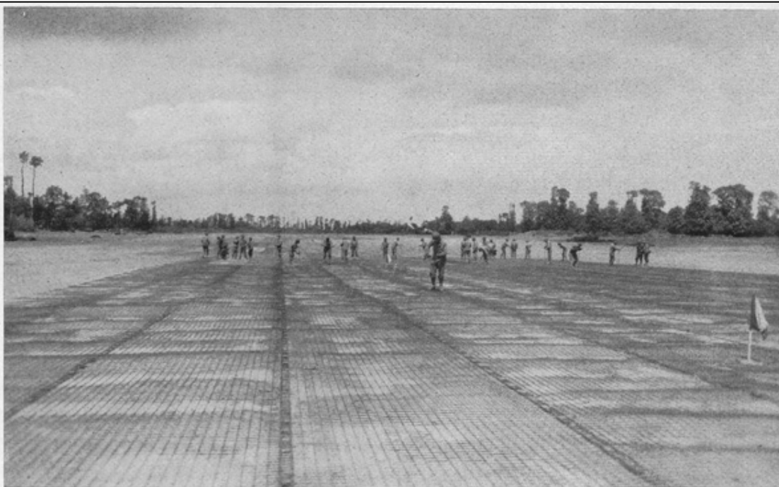
"Tightning-up" on the Cardonville Flying Strip of steel wire mesh. Normandy, June 1944
