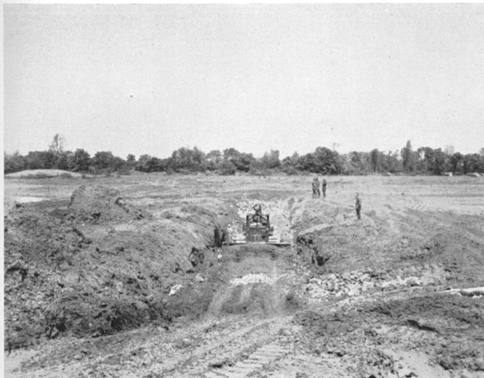
Cleaning out and refilling a big mud hole on the proposed runway area. Colleville-Sur-Mer, July 1944
