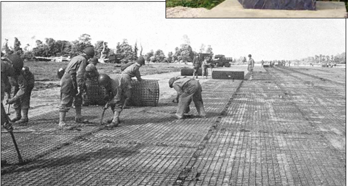
One of the airfields A-3 to A-8 (not otherwise identified), photographed on 17 June 1944, showing the kind of steel mesh construction used for many of the front-line airstrips.
