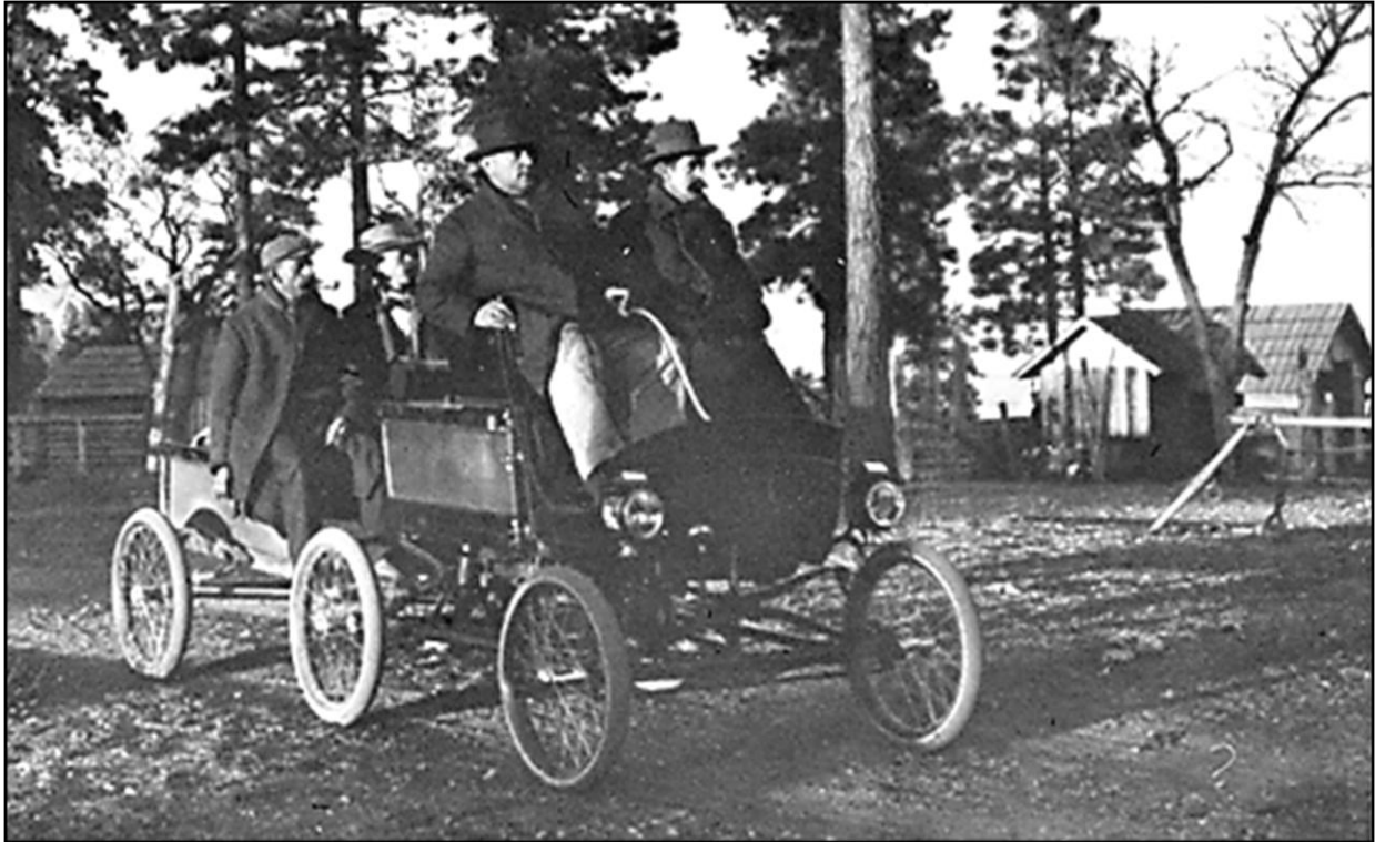
National Park Service, Grand Canyon National Park
